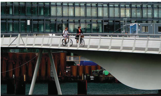
Above: Cycle and foot bridge, Copenhagen, Denmark
